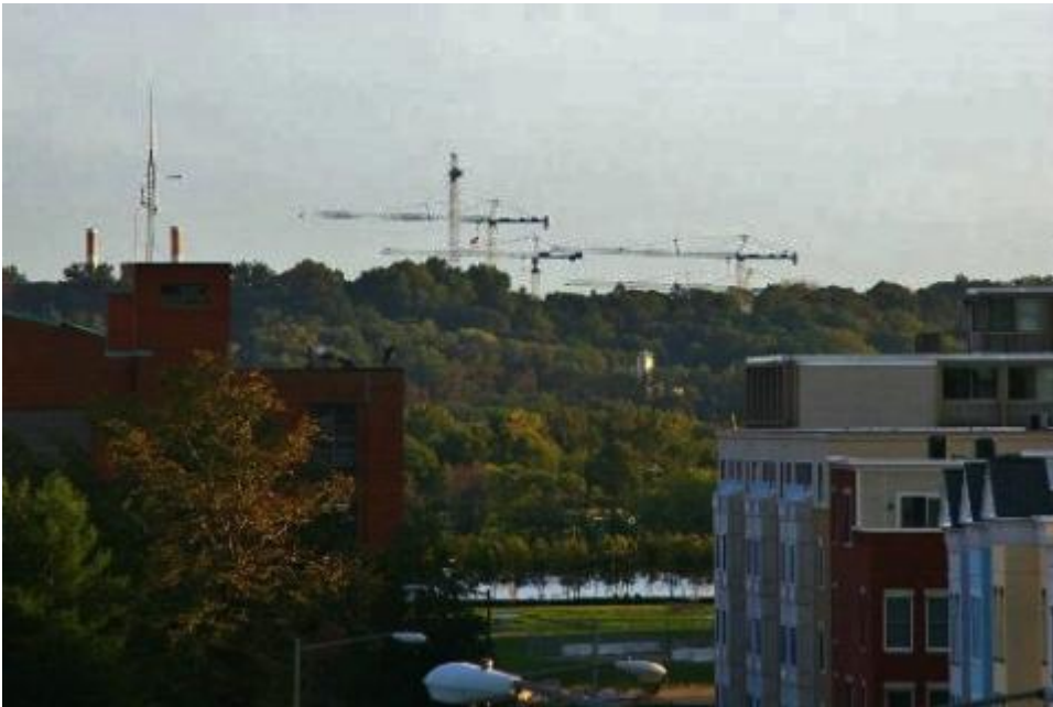
Construction cranes at U.S. Department of Homeland Security headquarters, Dec. 29, 2011 (Flickr/Tim Evanson)
