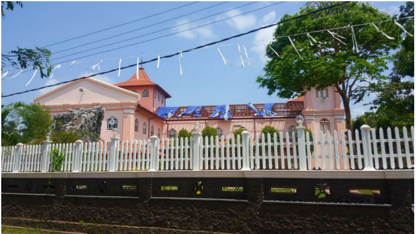
St. Sebastian's Church, Katuwapitiya, near Negombo, 23 miles north of Colombo, devastated by a bomb blast on April 21. (Thomas Scaria)
