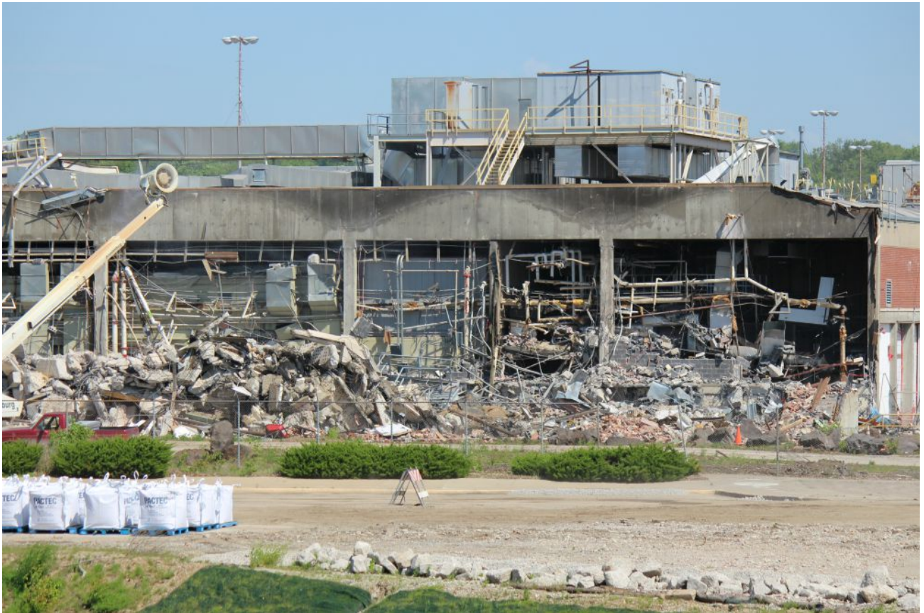
The Kansas City Plant, pictured May 16, 2019, is under demolition by a private developer. (NCR photo/Toni-Ann Ortiz)
