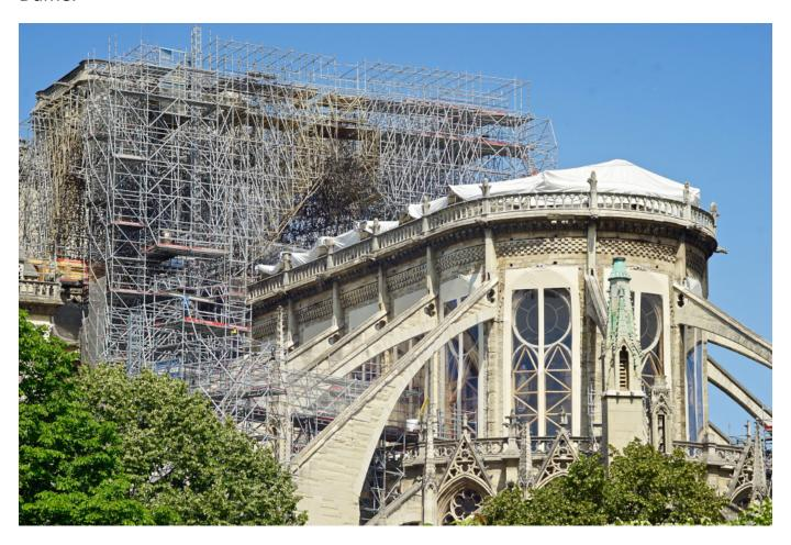
A view of the eastern end of Notre Dame Cathedral on June 15, 2019, showing the choir area where the glass has been removed from windows now stabilized by wooden supports. The white plastic sheeting on top protects replaces the burnedaway roof. The scaffolding above the cathedral was put up during the renovation work that led to the April 15 fire. (RNS/Tom Heneghan)
