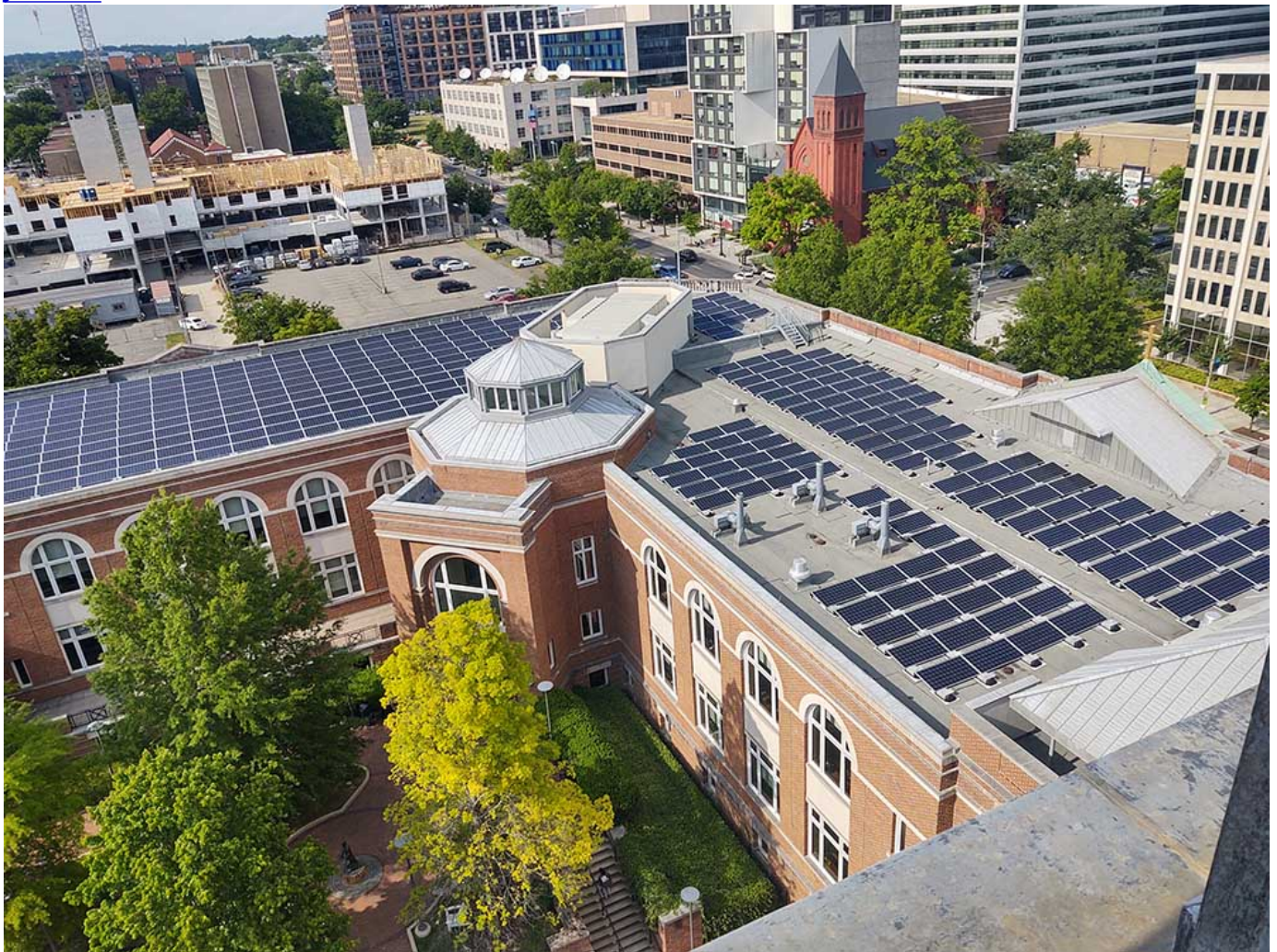
Solar panels on the roof of Gonzaga High School in Washington, D.C., on May 17 (RNS/Stephen Planning, SJ)
