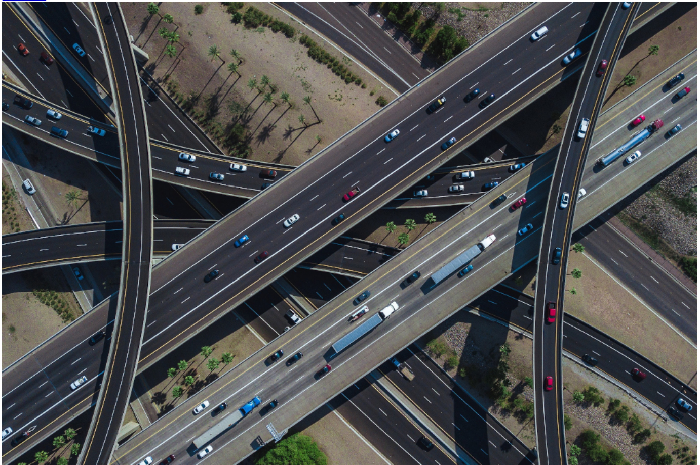
Vehicles travel along multiple layers of overpasses in Phoenix, Arizona. (Unsplash/Creative Commons/Jared Murray)
