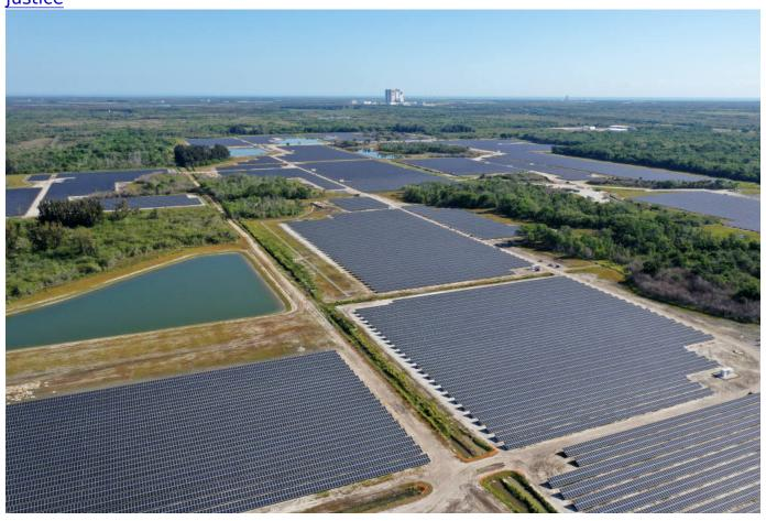
Florida Power and Light's new Discovery Solar Energy Center is a 74.5-megawatt solar site, spanning 491 acres at NASA's Kennedy Space Center in Florida. Its roughly 250,000 solar panels are expected to produce enough energy to power approximately 15,000 homes. (Flickr/NASA)
