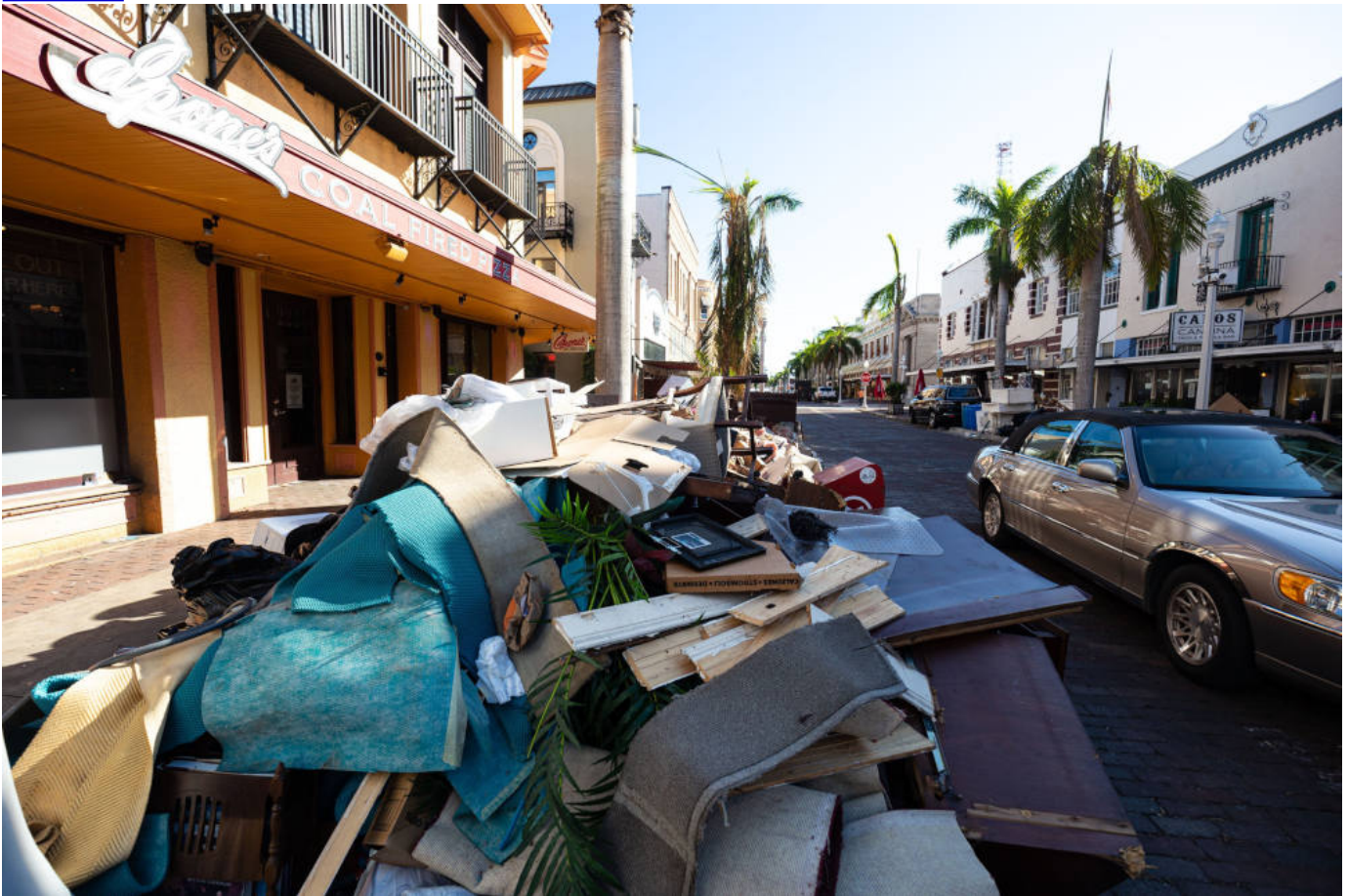
The downtown and waterfront areas of Fort Myers, Fla., show damage from the wind and storm surge Oct. 5, 2022, following Hurricane Ian. (CNS photo/Tom Tracy)
