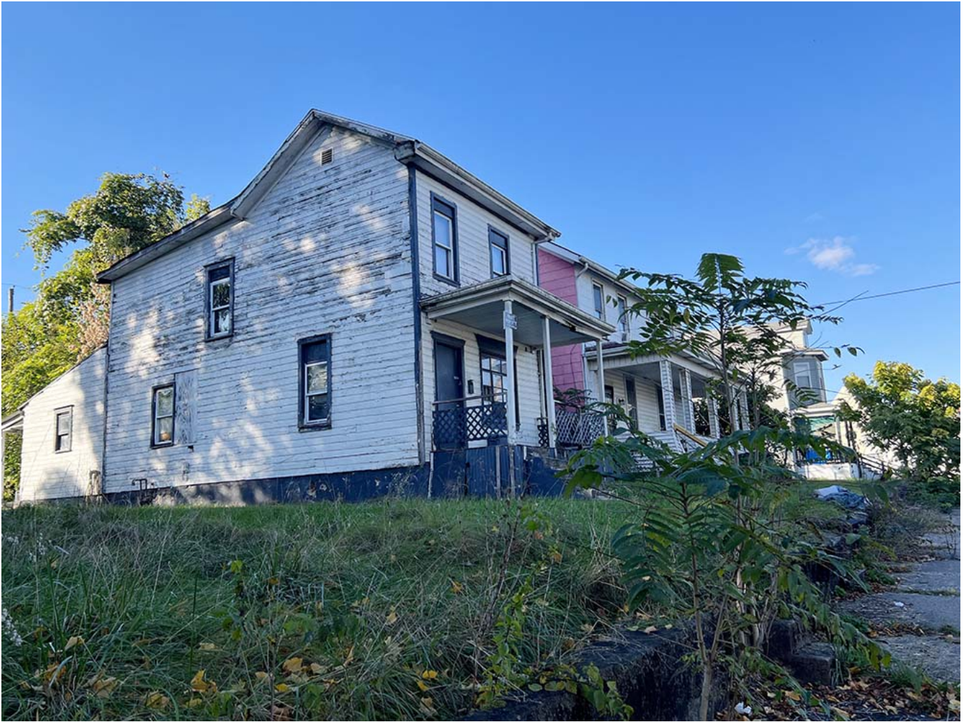
A rundown abandoned house in Steubenville, Ohio (NCR photo/Brian Fraga)
