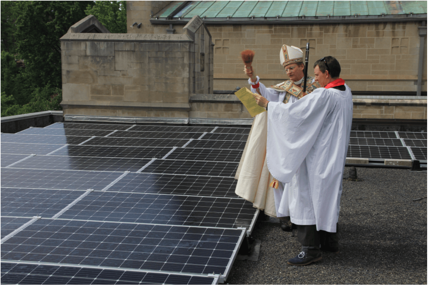
Former Pittsburgh Bishop Dorsey W.M. McConnell and Rev. Noah H. Evans bless the solar panels installed at St. Paul's Episcopal Church in Mt. Lebanon, Pennsylvania. (Courtesy St. Paul's Episcopal)
