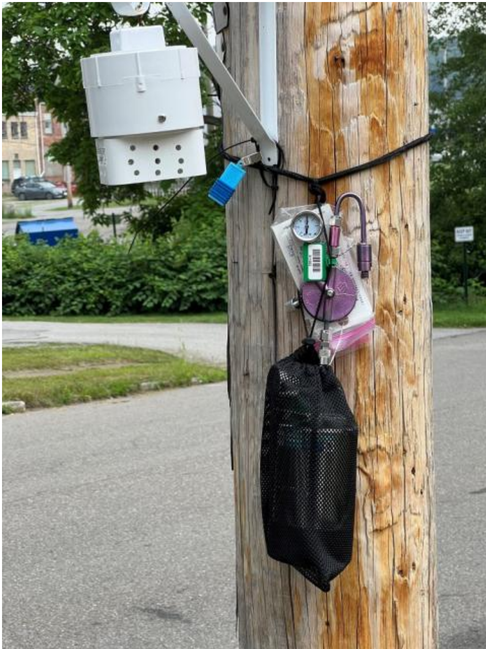
A passive air sampling device, blue near top, and other monitoring equipment on a utility pole in East Palestine, Ohio, July 17, 2023. (RNS photo/Kathryn Post)
