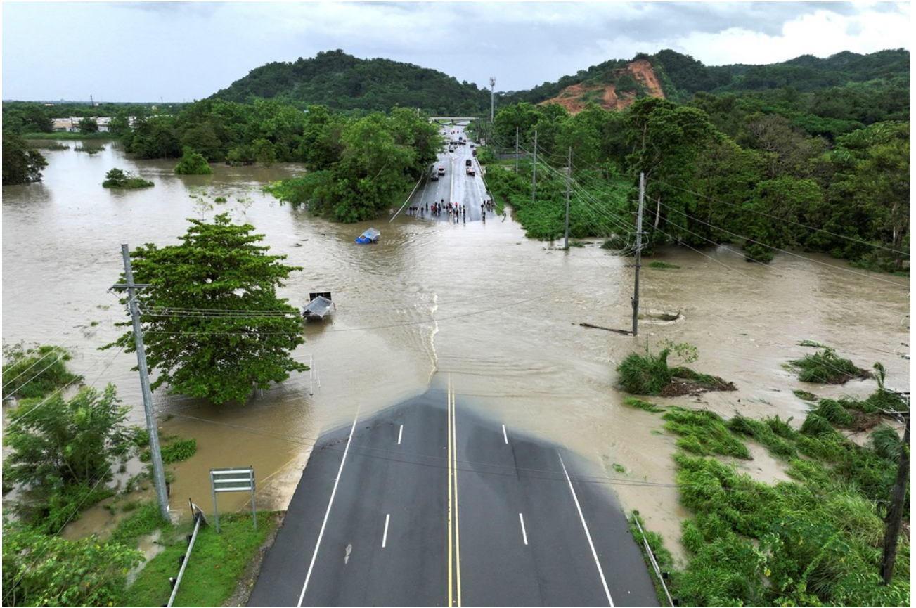
A drone view shows a bridge submerged by the flooded La Plata River in Toa Baja, Puerto Rico, in the aftermath of Hurricane Ernesto Aug. 14, 2024. Archbishop Roberto O. Gonzalez Nieves of San Juan suspended Masses and pastoral activities Aug. 13 and 14 as Ernesto battered Puerto Rico, leaving hundreds of thousands without power. (OSV News/Ricardo Arduengo, Reuters)
